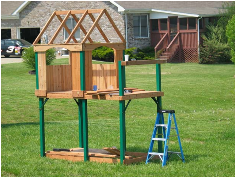
Figure 3. Partially Complete Swing Set (House Assembly)
