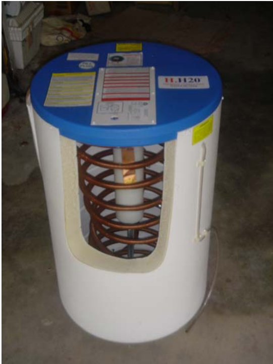
Figure 2. Harris Water Heater Cut-Away
